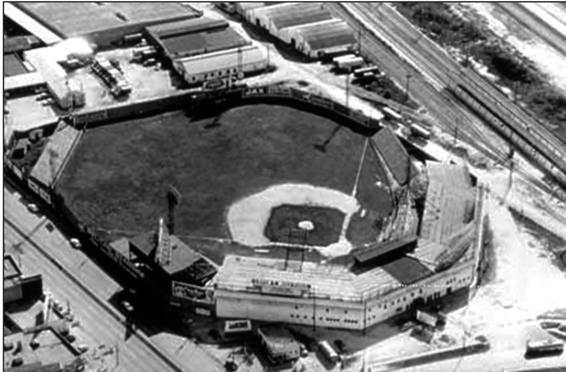
Pelican Stadium New Orleans, Louisiana
