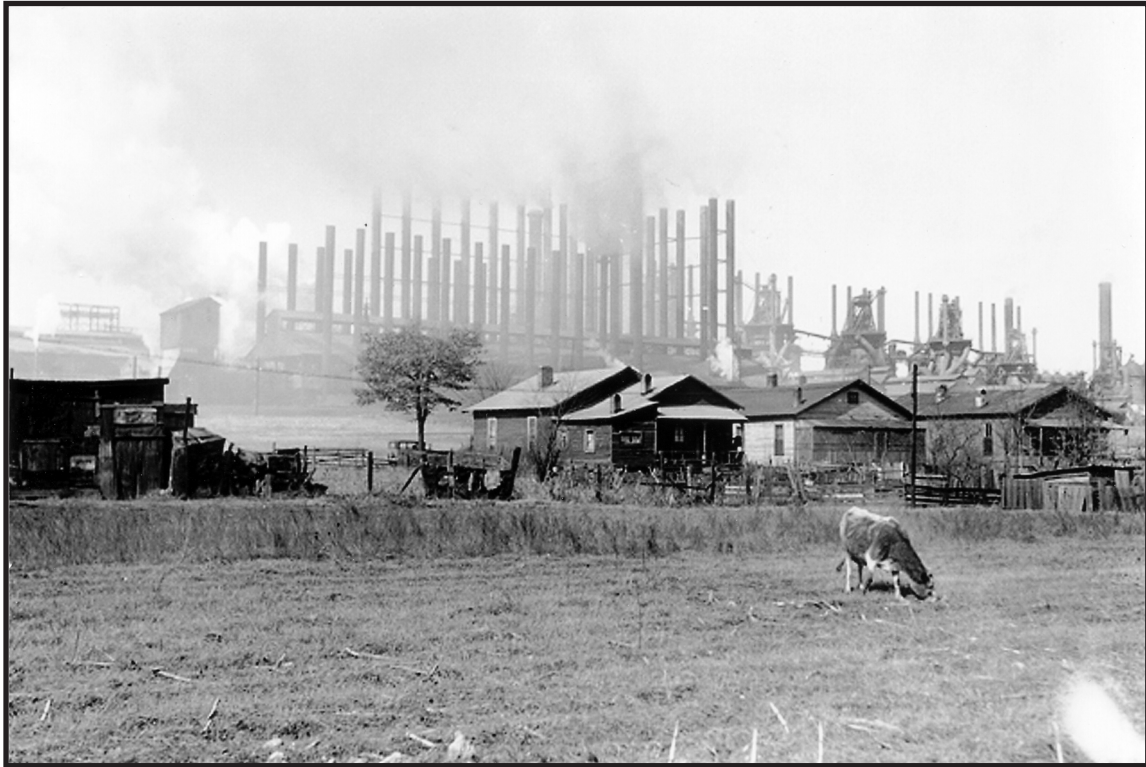
ACIPCO Plant Birmingham, Alabama (Late 1930's)
