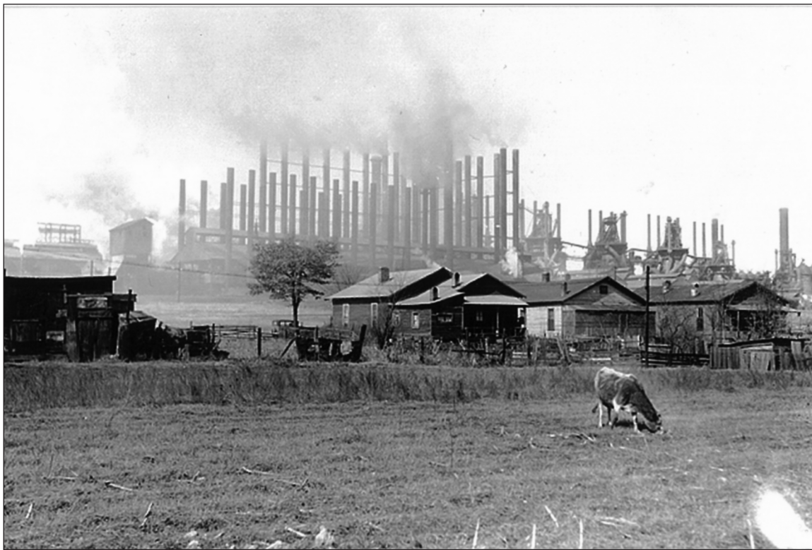
ACIPCO Plant (c. 1930's) Birmingham, Alabama
